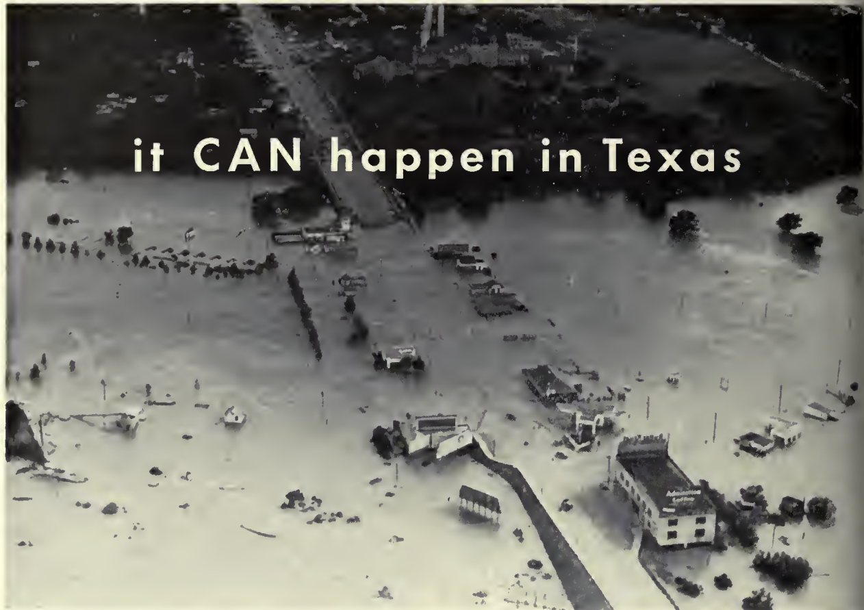
THE FLOOD OF JUNE 15, 1935.—Looking south along Congress Avenue, Austin, Texas, with the Colorado River flooding the
